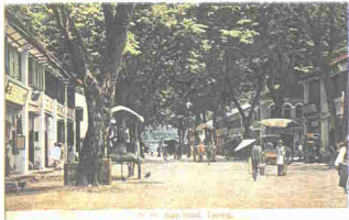
Main Road, Taiping
